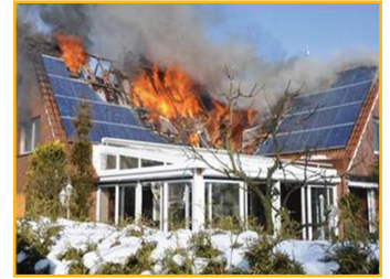
Eliminating of any flammable materials from the base structure of a module greatly reduces the fire hazard and fume generation at high temperature.
