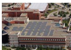
On-grid commercial/ industrial roof-tops
