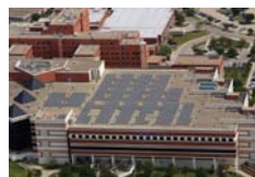
On-grid commercial/ industrial roof-tops
