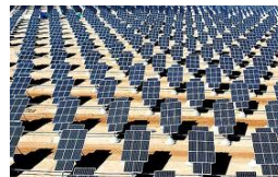
Solar Power plants
