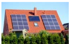
On-grid residential roof-tops
