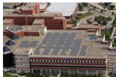
On-grid commercial/ industrial roof-tops
